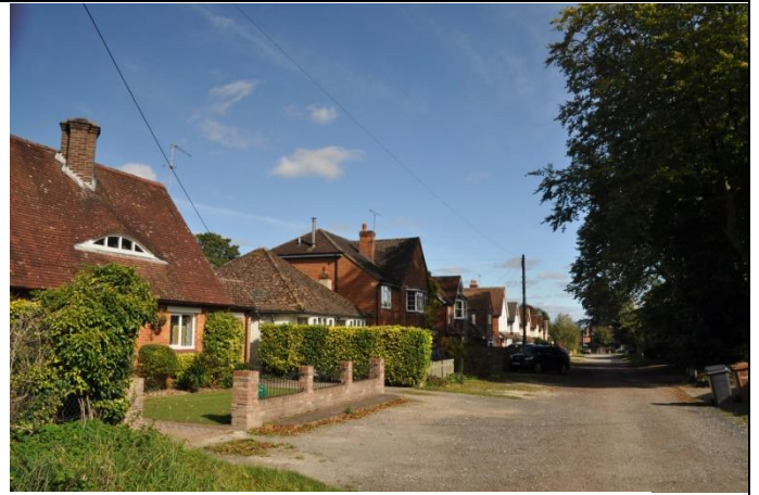
Figure 1A -2 View north-east of the western half of the area showing distinctive eyebrow dormer window in the foreground
