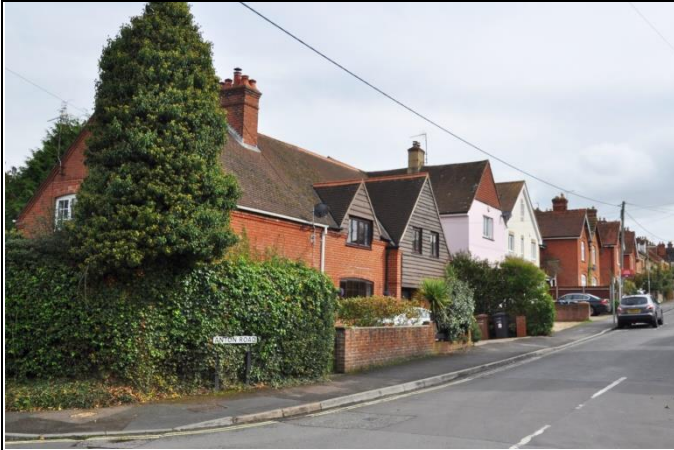
Figure 2B -1 Looking south east at north western corner
