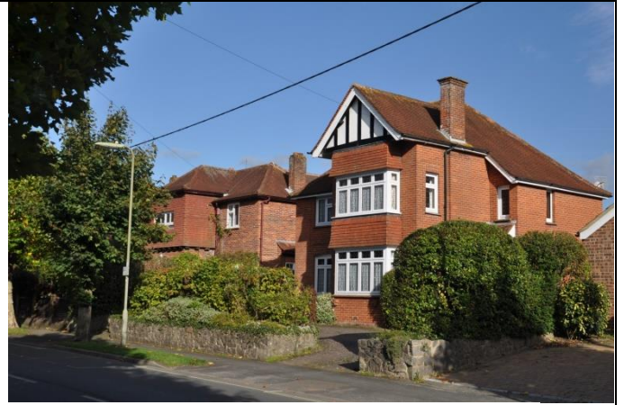
Figure 1B-2 View north east. Showing houses featuring tile hanging to the bays
