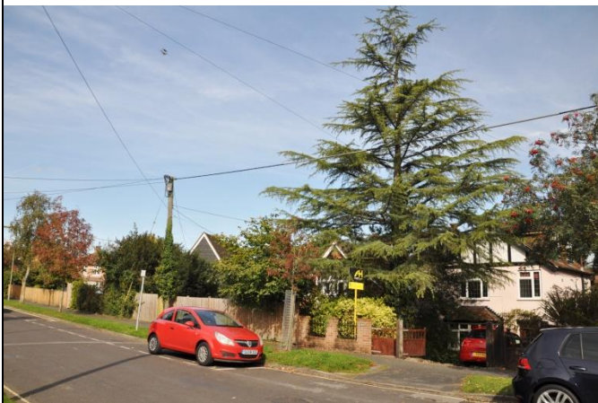
Figure 1C-3 Looking north west towards properties along the north side at the western entrance to Bishop's Way. The fall away from the road towards the houses leads to the buildings on the north side being less dominant in the streetscene
