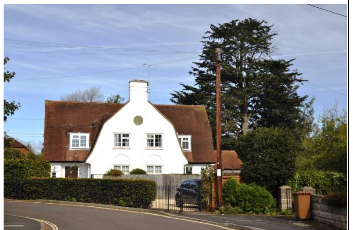
Figure 1E-6 View from north west from beyond the south eastern end of the area. Note the distinct Dutch barn roof of this building, 'South Croye'. The central section, adorned by a gable façade turned towards the street, with its cream painted render, forms a distinctive and attractive gateway feature to the area
