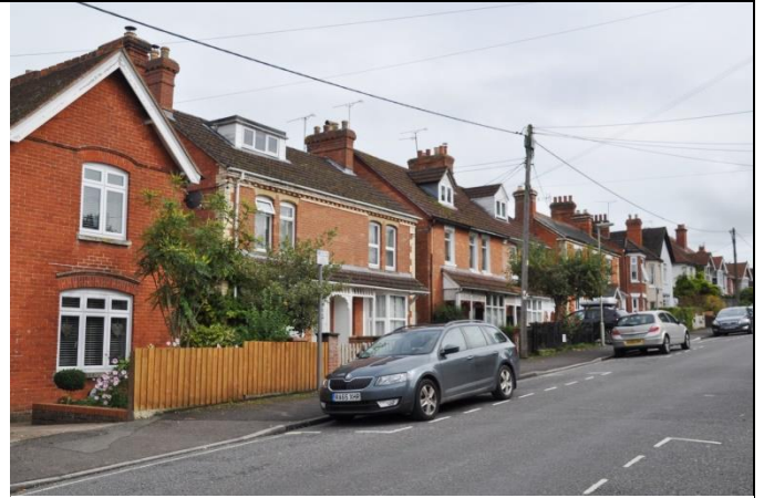
Figure 2B -2 View south east looking towards the main group of Edwardian buildings
